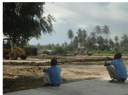
New school construction
